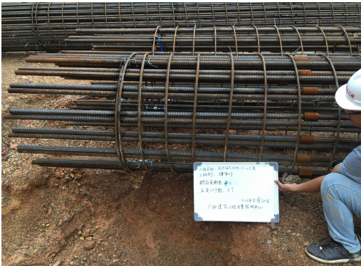
图2 基桩内力测试传感器安装 Fig.2 Sensor installation of pile internal force test
